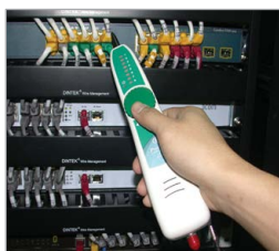
Copper cabling detecting
