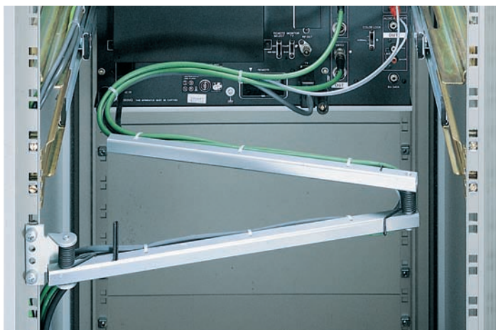
Cable support with return spring
