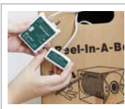
RJ11 cable test
