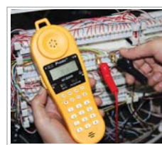
Telephone line testing
