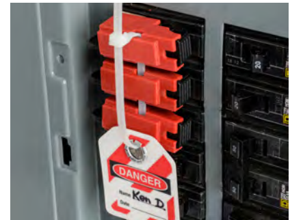
120V breaker lockout devices fit on breakers next to each other, enabling multiple tagouts at one time
