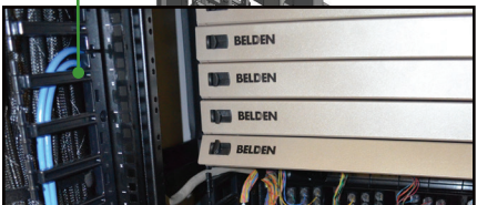
Vertical Manager shown in enclosure
